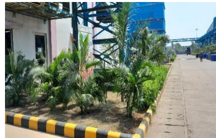
Production Plant Area
